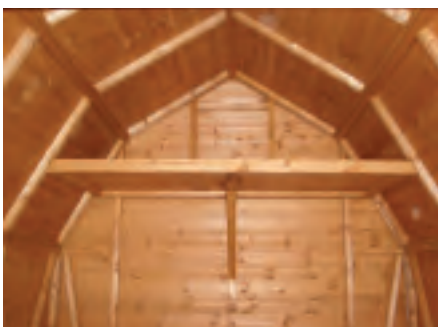
Internal roof and shelf
